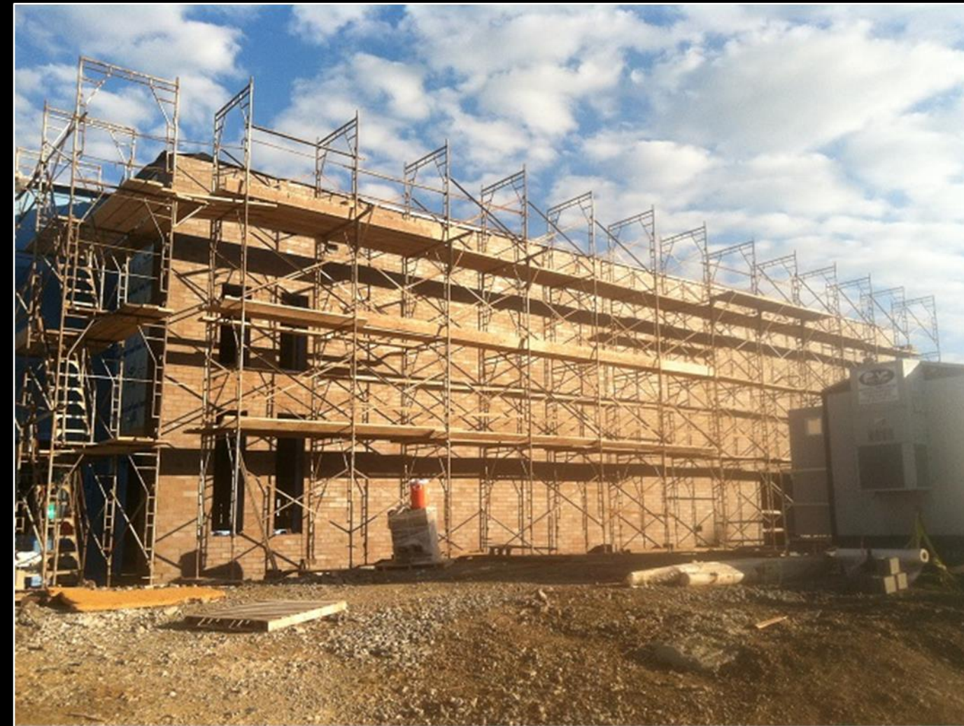
Scaffolding Congestion – Area E North Elevation
