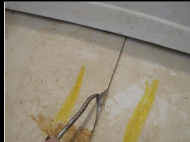
Failed TPO at CWNCHS
